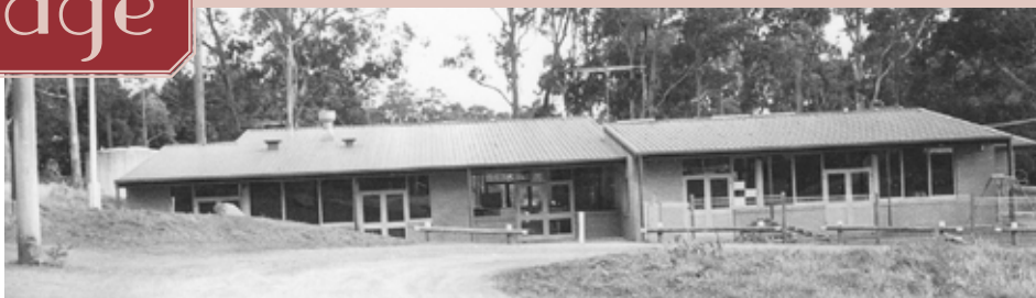
Above: New Community Centre. Below: Opening in the Community Centre Hall.
